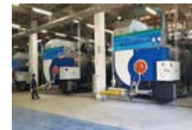
Installation of ultra-low NOx boiler
